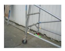
Lay out the required equipment for the base of the mobile in a safe area. Tower scaffold (no castors) need to be erected in the position that it is to be used.
