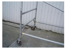
Install baseplates/jacks/castors into ends of End Frames and stand upright. Attach yellows in position depicted in picture from one frame to the other. Install blue braces on each side running opposite to each other.
