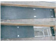
The pictures above shows the "Fully Hinged Access Deck" in the "closed" position at the top and the "open" position at the bottom.
