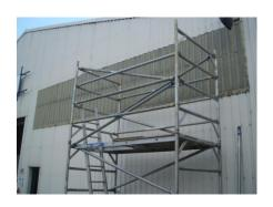
If there is Two Working Platforms the lower Working Platform MUST have three (3) yellows installed as shown to meet the minimum Guardrail height and a ladder installed protruding through the Access Deck.
