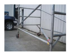
Install red plan brace diagonally across frames if a Working Platform is equal to or more than 3m from supporting structure.
