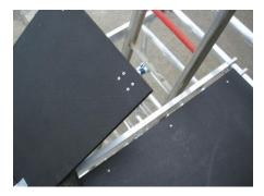
The above picture depicts the correct placement of the ladder when placed through the Access Deck.
