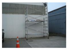
Install End Frames onto each end and attach blue braces as depicted in the supplied picture for the height of Mobile or Tower that you are erecting.
