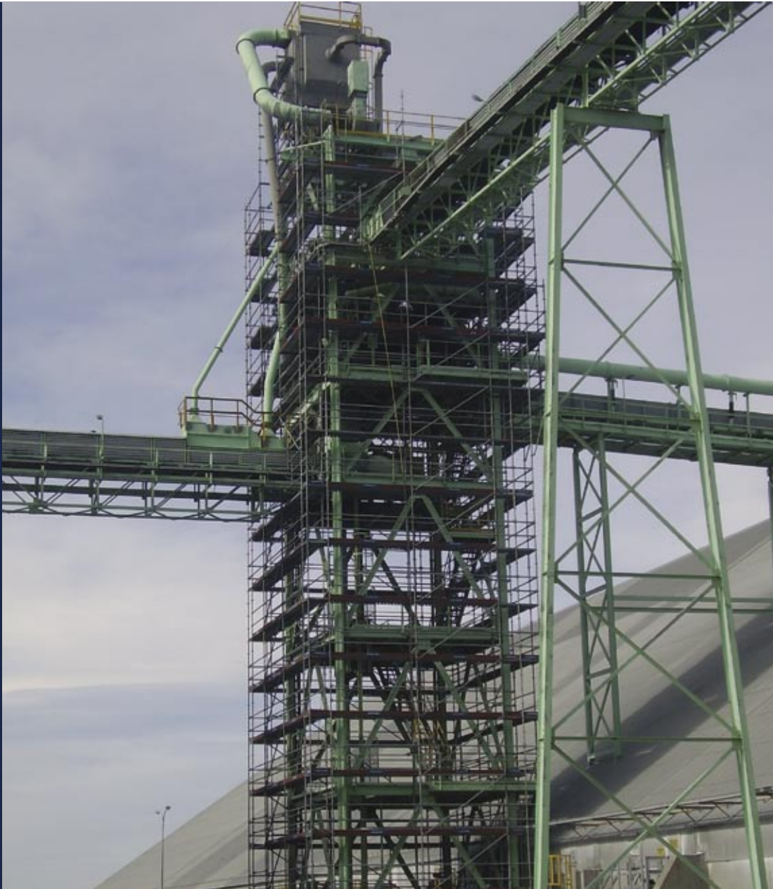
NZAS T1A tower upgrade for Pneumatic Contractors
