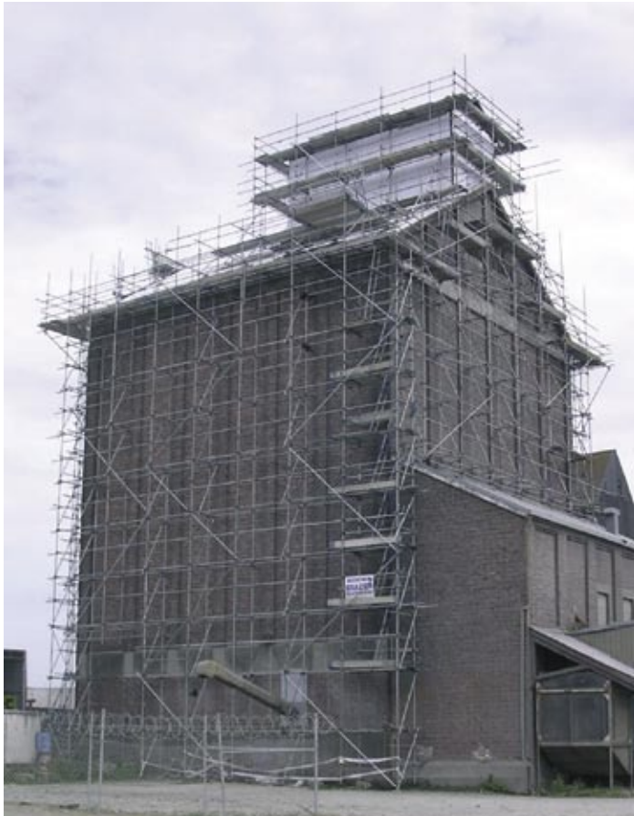
Addington Grain Store is prepared for a new roof
